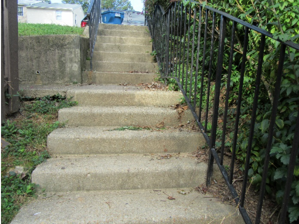
Concrete stairs overview
