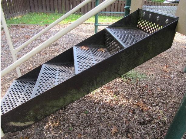
Finish deterioration – Note: Whipple Court
