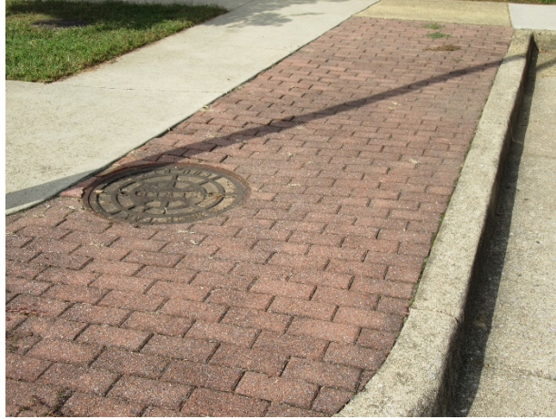
Masonry pavers overview
