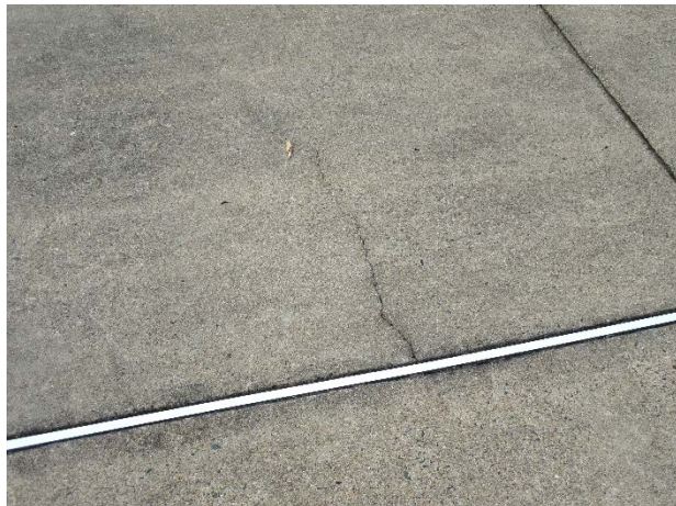
Concrete crack
