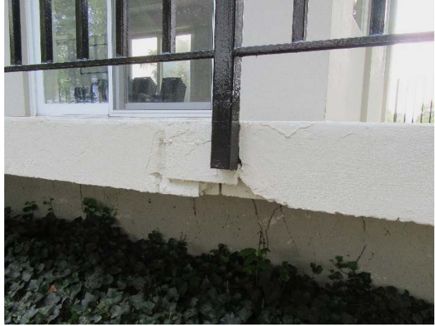
Concrete deck deterioration
