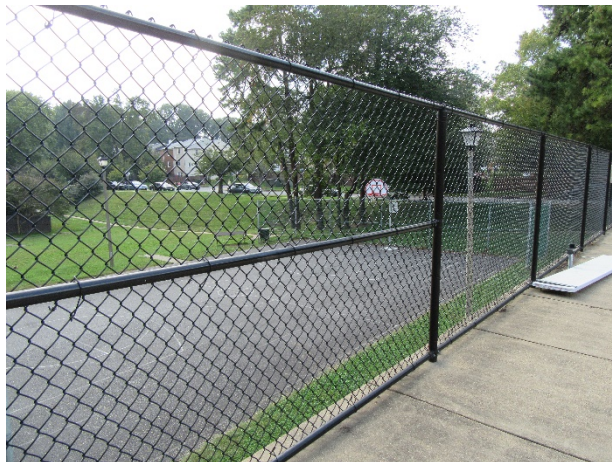
Chain link fence overview
