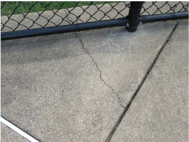
Concrete crack
