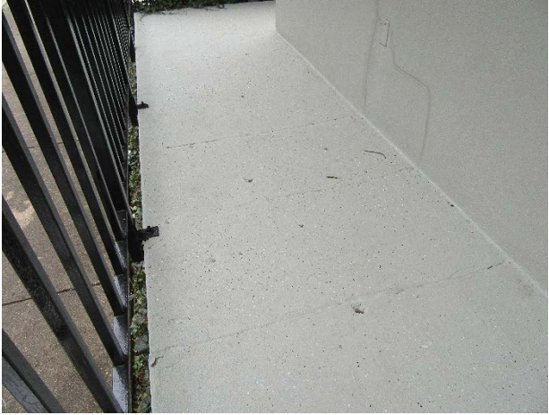
Concrete deck overview – Note: previous repairs
