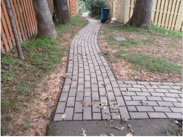
Permeable paver walkway at Breckenridge Court
