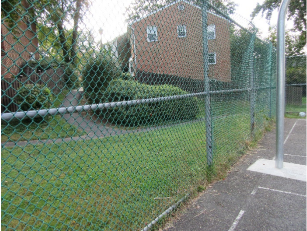
Chain link fence overview
