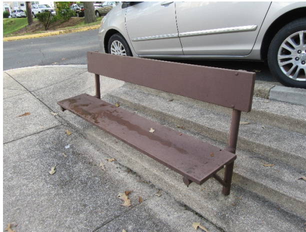
Site furniture overview
