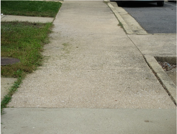
Concrete sidewalk overview
