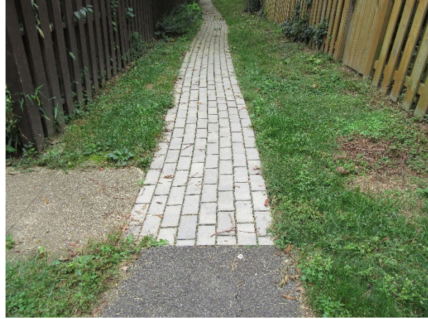
Permeable paver walkway at Breckenridge Court
