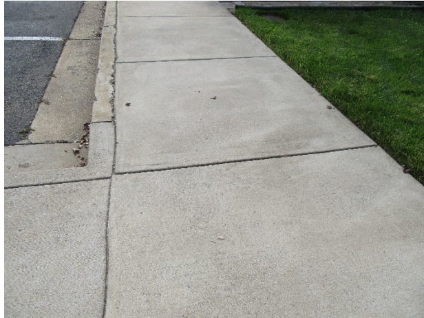
Concrete sidewalk overview
