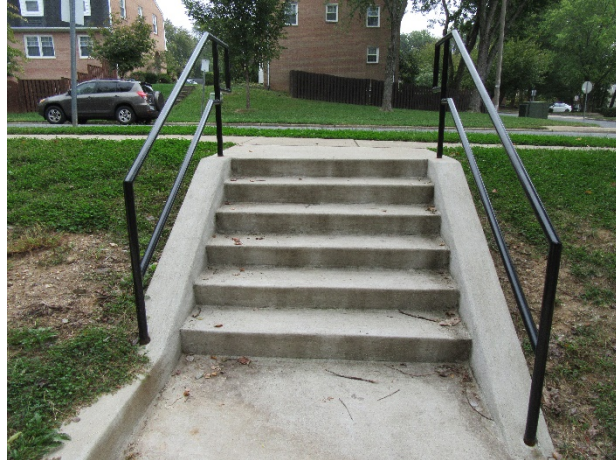
Concrete stairs overview
