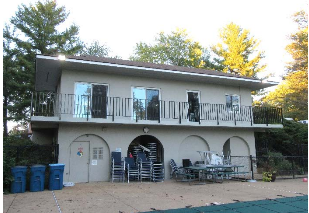
Rear elevation overview
