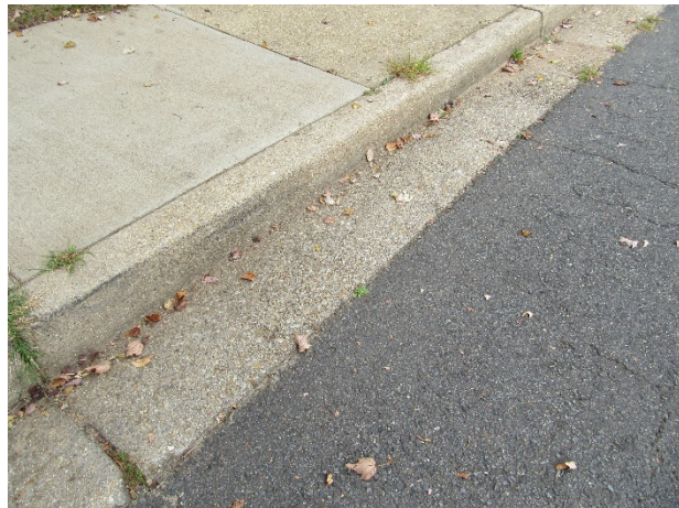
Concrete curb and gutter overview
