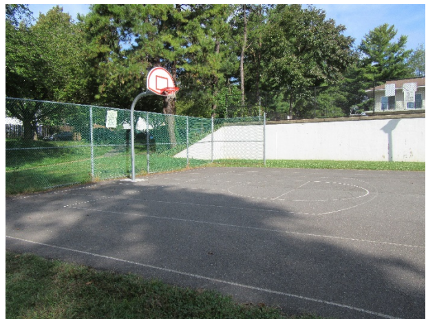
Asphalt pavement basketball court overview
