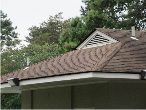
Asphalt shingle roof overview – Note: stains
