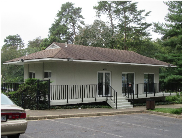
Front and partial side elevation overview
