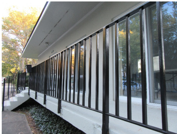
Metal deck railing overview
