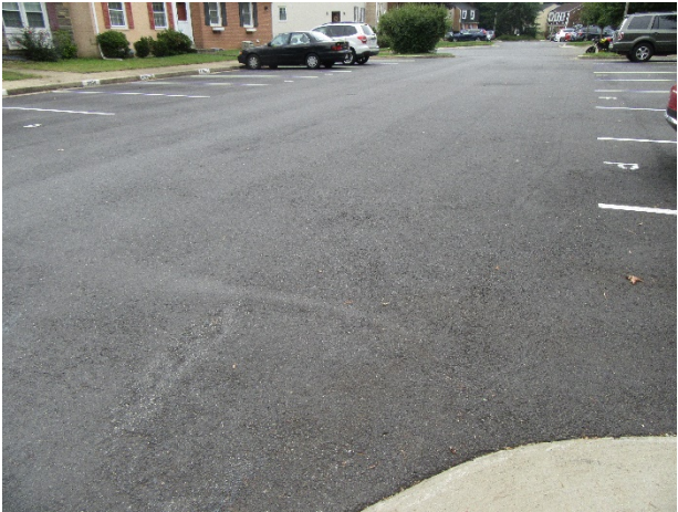
Asphalt pavement overview – Note: Breckenridge Court
