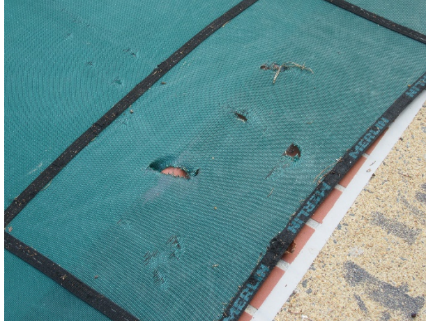
Vinyl cover damage – Note: main pool
