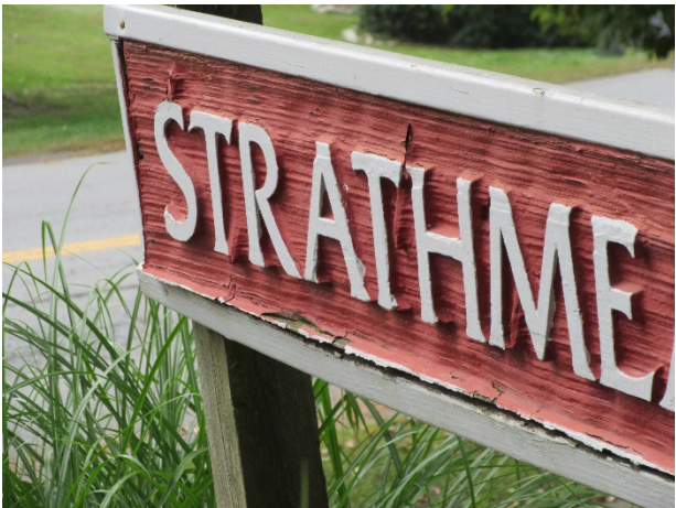
Paint finish and sign deterioration
