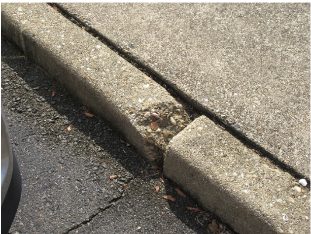
Curb spall and gutter crack
