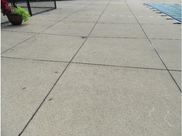
Concrete pool deck overview
