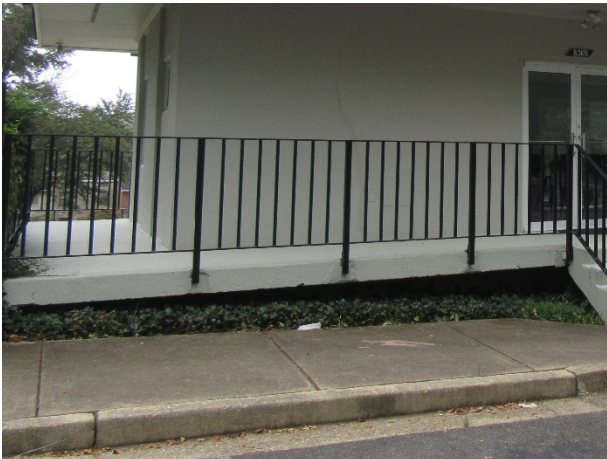
Concrete deck and railing overview
